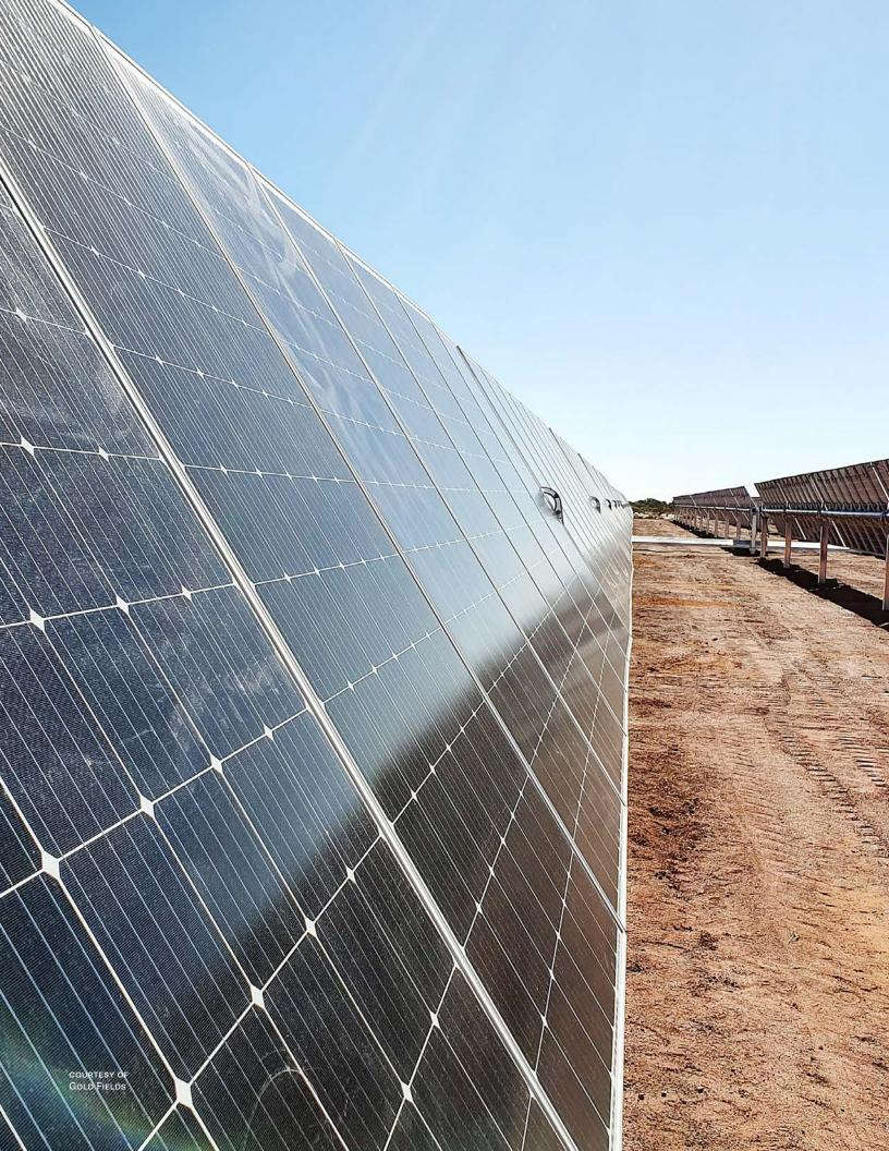
10,000-panel solar farm contributing 4 MW, a 13 MW/4MWh Battery Energy Storage System and a 16MW gas engine power station to underpin supply when required. The combined project is initially forecast to provide 55 - 60% of the mine's electricity needs during daytime hours with potential to meet almost all electricity requirements at certain times.
