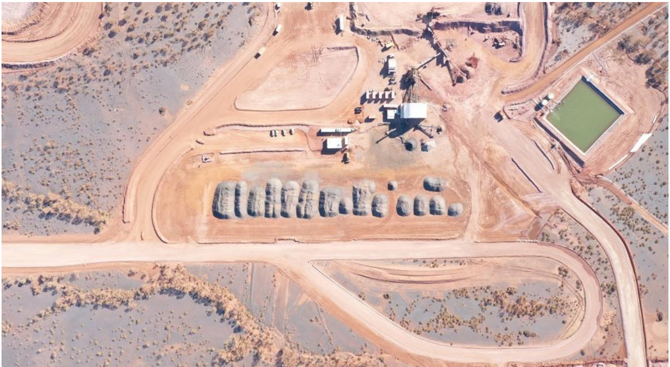
Completed Stage 1 operation at the Butcherbird mine site in Western Australia
